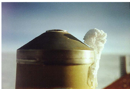
FIG. 6. (Color online) Vapor heated hollow exhaust stack. Photo was taken when station was opened showing that ice formation was minimized on this exhaust stack and the ice did not plug up the exhaust orifice on the top of the stack.
