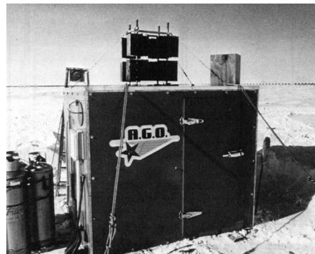
FIG. 3. Prototype Automatic Geophysical Observatory at the South Pole ca. 1983.
