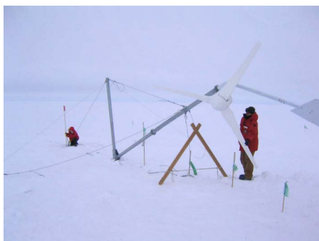
FIG. 18. (Color online) AWP turbine installation at a field site. The WT is attached to the 20 ft pole and then winched into place.
