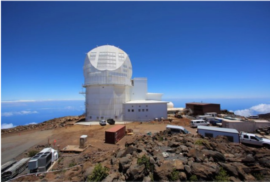
DKIST - a 4-m solar optical/IR telescope
